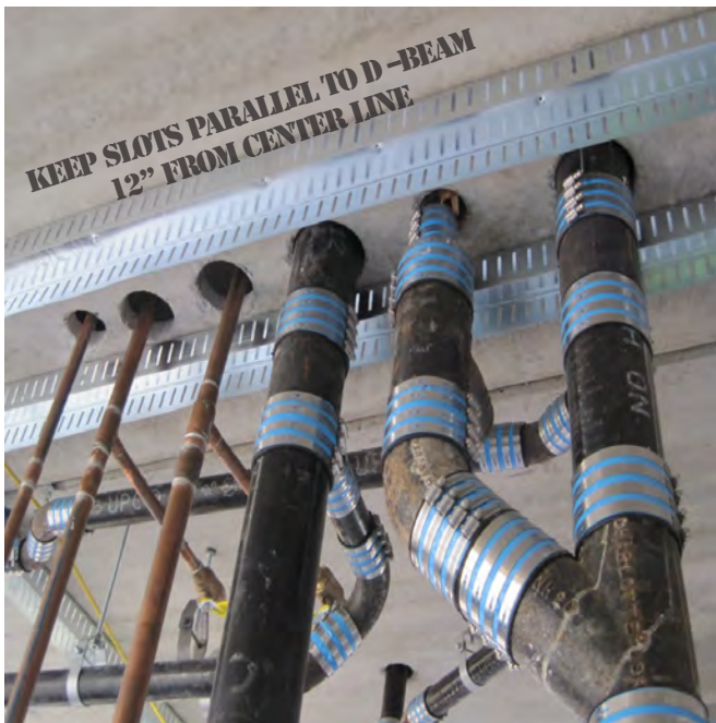
Rebar is for shrinkage so it can be cut during coring. Plank pre-stressing strands are bonded so if cut, the pre-stressing force is not compromised.
