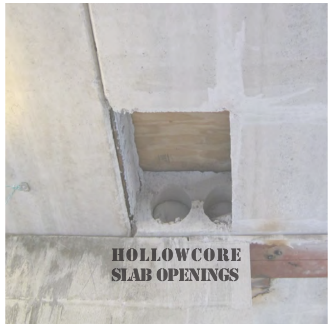
A wide variety of opening sizes and configurations can be accommodated ranging from "large" openings (>10-inches) to small core drills. Most common large openings include: HVAC, plumbing and electrical chases, hatch access at roof, trash chutes and skylights.
